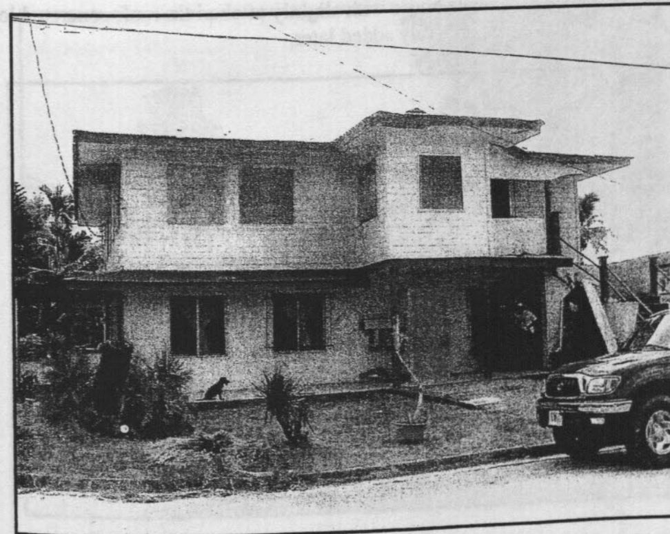
Photo 9. Agat: two story house with tin roof, eaves, and stairs to second floor. The first floor has concrete walls while the second floor walls have horizontal wood siding.
